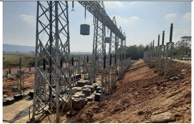
Earth cutting and Surface levelling at 220/ 132 kV Amingaon GIS S/S
