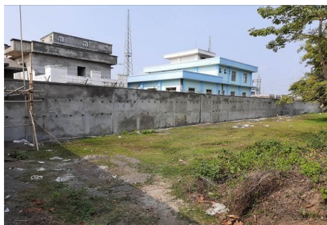
RRM Wall at 220/ 132 kV Amingaon GIS S/S and 132/ 33 kV Tezpur S/s
