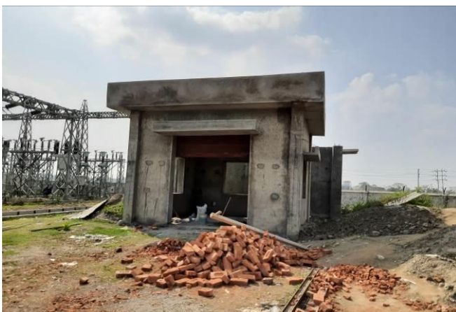
Fire Fighting Pump House, Water Tank, Cable Trench at 132/33 kV Hazo S/S
