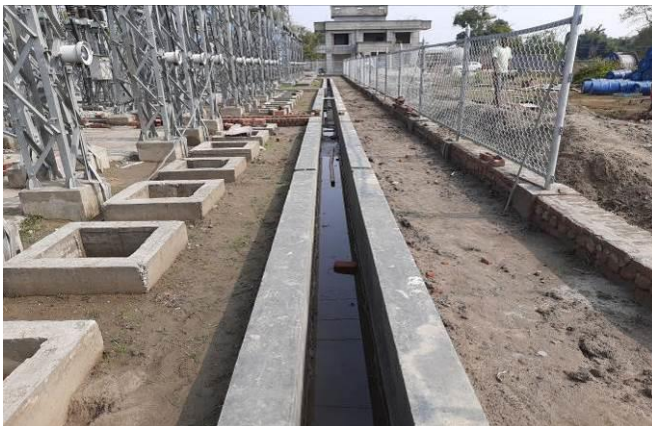
Drainage within the 132/33 kV Tezpur S/S
