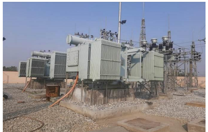
Oil Spill Containment Systems at 33/11 kV Sesa and Harisingha S/S
