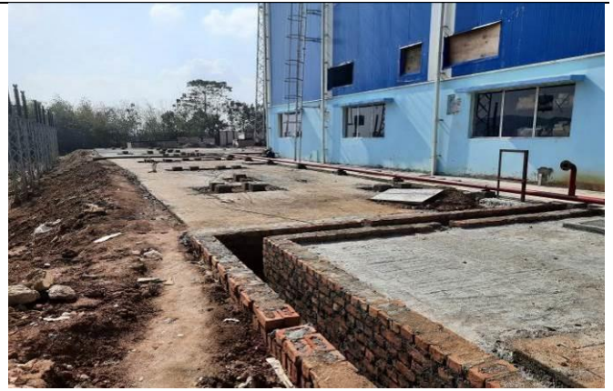
Drainage within the 220/132 kV Amingaon GIS S/S
