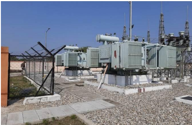
Oil Spill Containment Systems at 33/11 kV Ramdiya and Domdoma-Hazo S/S
