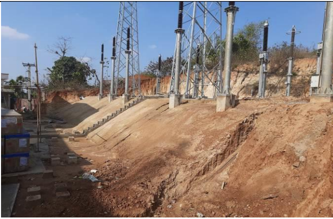
Earth cutting and Surface levelling at 220/ 132 kV Amingaon GIS S/S
