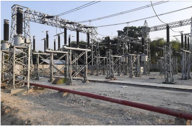
Water Spray System at 132/33 kV Tangla S/S
