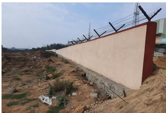
RRM Wall at 220/ 132 kV Amingaon GIS S/S and 132/ 33 kV Tezpur S/s
