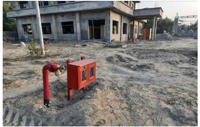
Water Spray System at 132/33 kV Tangla S/S
