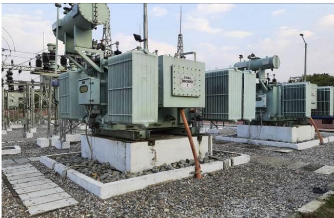
Oil Spill Containment Systems at 33/11 kV Sesa and Harisingha S/S
